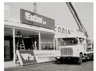
Eastland Bank branch at the Walnut Hill Plaza
