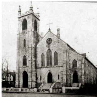
St. Charles Church after the fire
