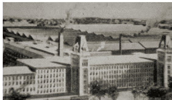
Social Mill complex after the fire
