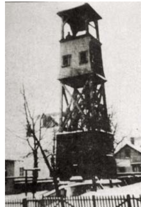
Boyden Street Fire Tower
