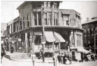
Edwards Block after the fire
